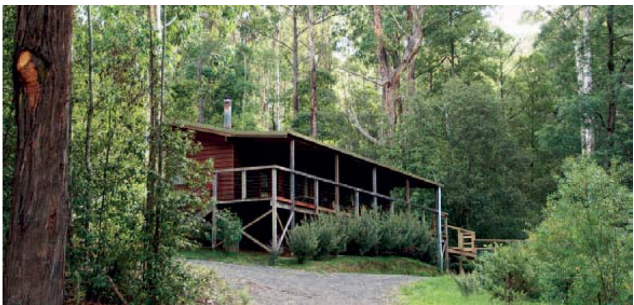
Radiant heat can ignite a house
