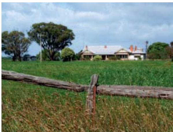
Home located in open environment
